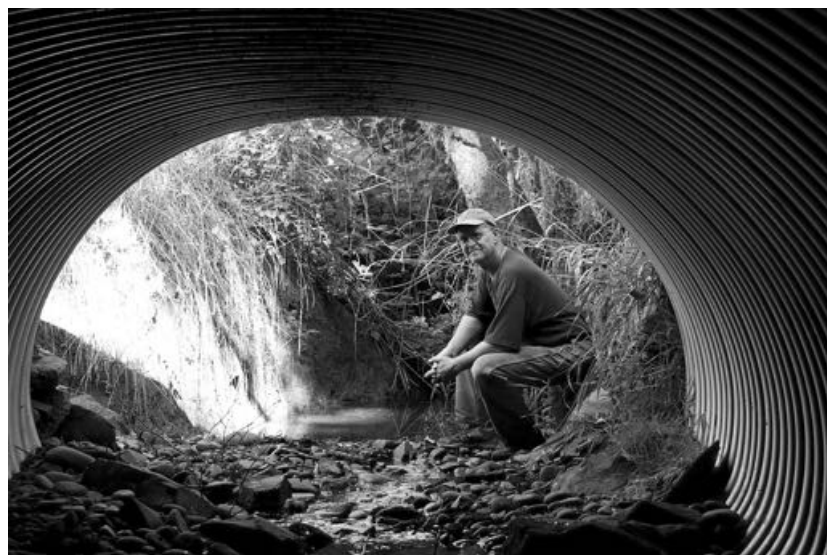
At Winter Green Farm, Jack Gray designed culverts with gentle angles and rocky beds to mimic natural creek contours to help fish migrate.
